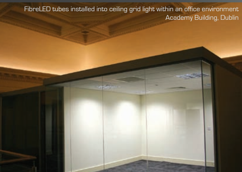
FibreLED tubes installed into Ceiling Grid lights in an office environment HSE HQ Swords, Dublin
