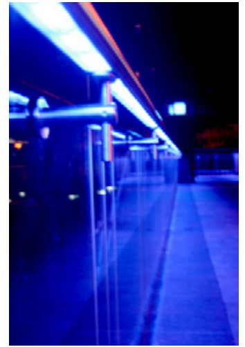
FL Stripline within handrail
