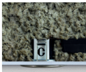
Blown insulation
