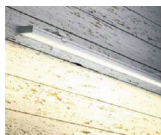
SURFACE B installation
